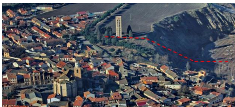
Figure 30. Aerial photograph of the natural slope.
