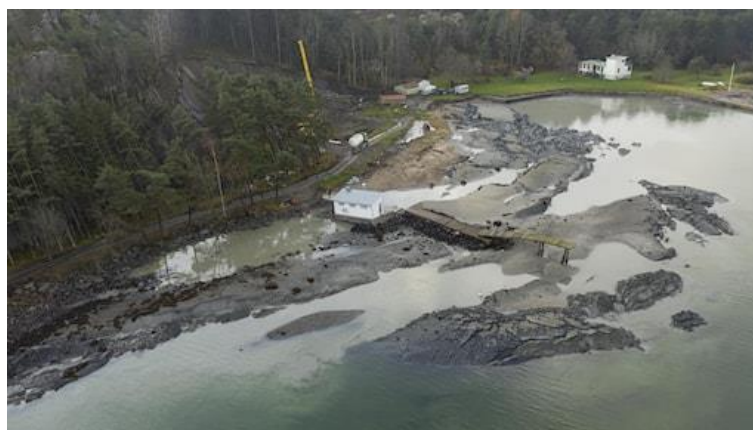
Figure 39. Example of landslide at Göta Älv river.
