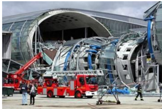
Figure 2-4. Collapse of Terminal 2E of the Charles de Gaulle Airport, Paris, France (2004) 7
