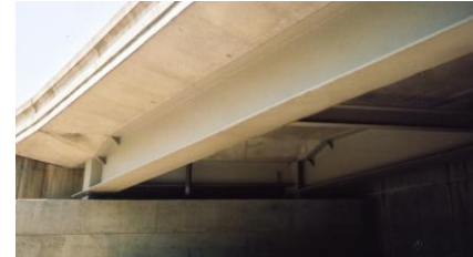
Composite steel-concrete bridges
