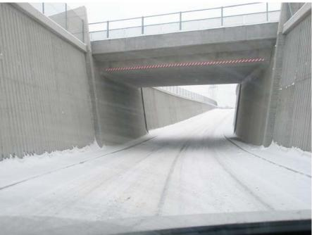
Integral concrete bridge Overall length: 14,0 m Superstructure: Concrete slab, thickness 1,10 m
