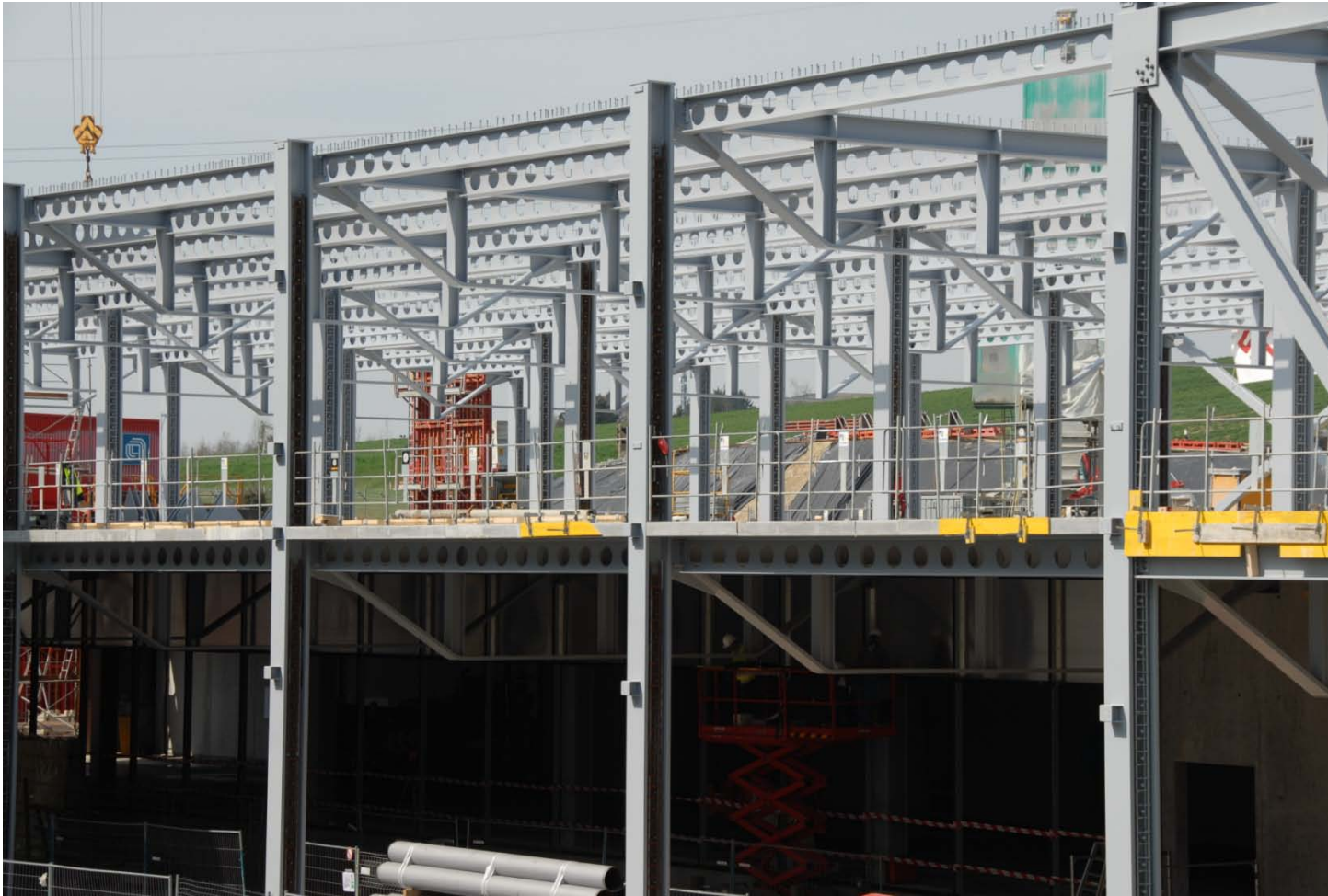
Braun Building in Crissier Production of Medical Material
