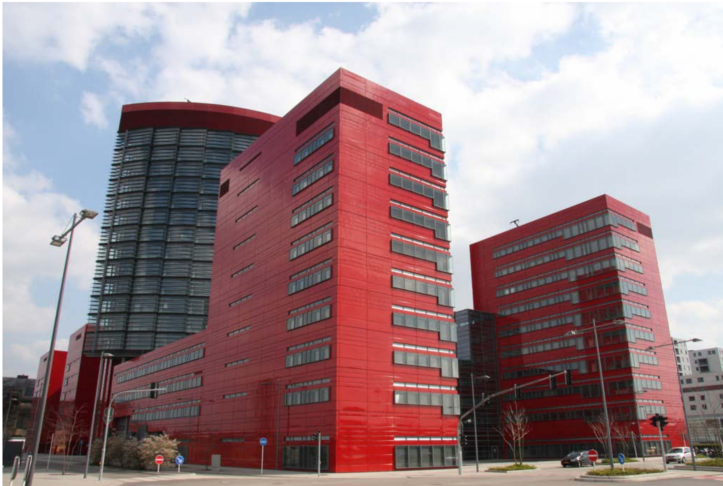
Dexia-Bil in Esch sur Alzette Office Building
