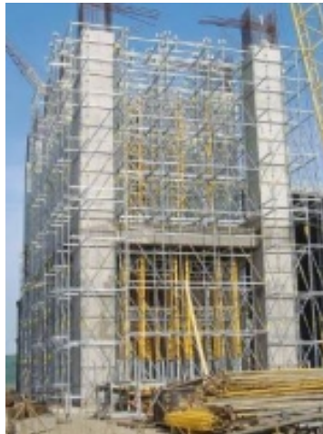
Geometry of the partially completed resisting structure
