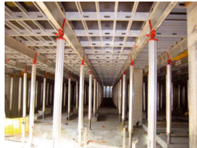
Resistance of the lower floor, which has not necessarily attained its full strength.
