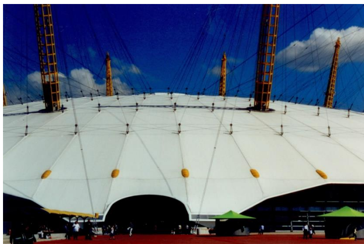
Figure 1-15 Shortening of aerial ties [© M. Mollaert]
