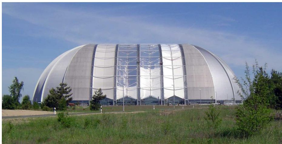
Figure 1-14 Cargolifter Airship Hangar [© formTL]
