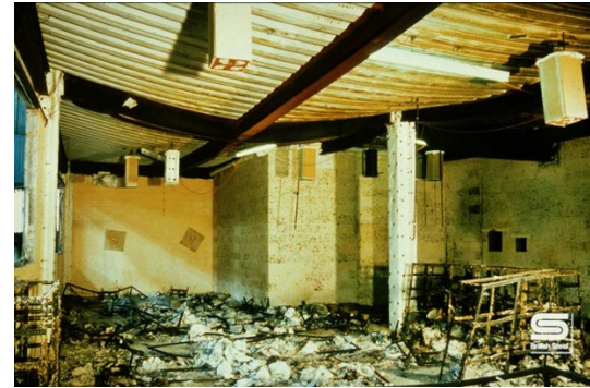
Source: Behaviour of multi-storey, steel framed building subjected to natural fire effects: Final report (2002)
