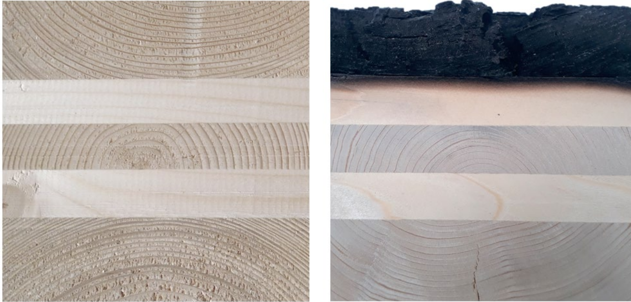
Cross laminated timber before (left) and after (right) a 30 minutes fire occasion
