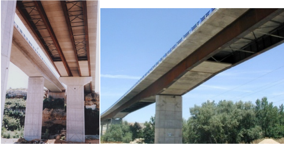
Fig. 6.10 Two examples of road composite bridges with double composite action in hogging areas
