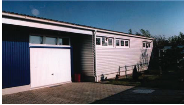
Figure 4.75 WSMS after completion ( two different span modules coupled)
