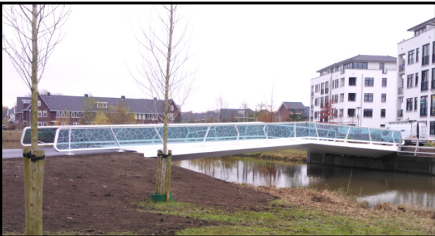
'Bronlibelle' Bridge in Harderwijk, the Netherlands. A 6.3 m wide, 22 m long GFRP bicycle / footbridge connecting two new districts of Harderwijk. At the same time unlocking an efficient route for heavy emergency vehicles (e.g. firetrucks). The bridge deck is made by applying the vacuum infusion technology, thus providing excellent properties with desired freedom for design. The bridge is designed according to CUR96, EN 1990 and EN 1991. Architectural and preliminary design by Royal HaskoningDHV. Engineering, production and installation by Delft Infra Composites B.V.
