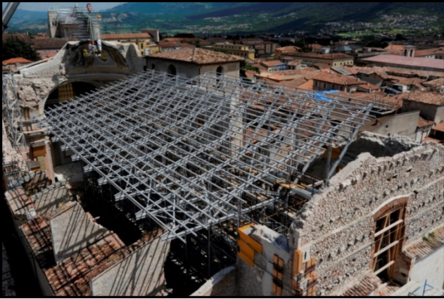
S. Maria Paganica Church, L'Aquila (Italy). Replacing the roof of the church damaged by the earthquake of April 2009. GFRP pultruded members. Designers: prof. Salvatore Russo, ing. Alessandro Adilardi. Contractor: Top Glass S.p.A, Osnago (LC), 2010.
