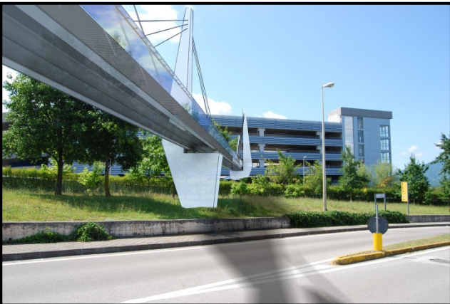
Salerno (Italy). Pedestrian bridge at the University of Salerno. Length: 148 m; main span: 37 m. GFRP pultruded I-beam. The deck is made of GFRP sandwich panels. Designer: prof. Luciano Feo, 2014 (In construction).
