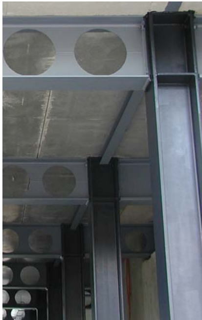
Figure 8-3: Beam to column connection
