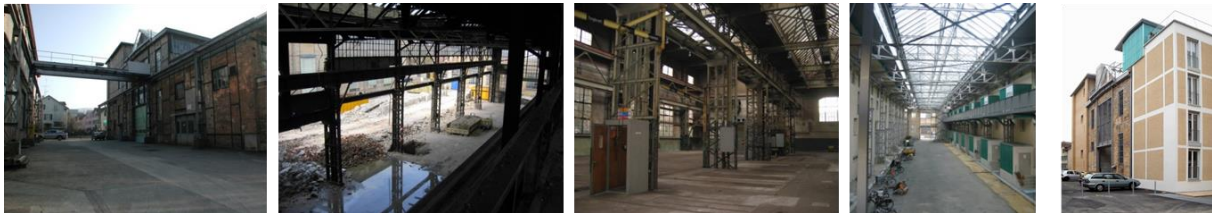
Figure 7.1 Reintegration of an existing industrial building into a new residential development area
