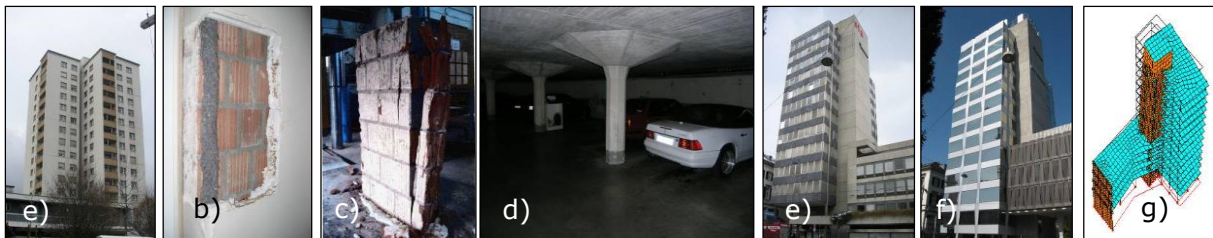
Figure 7.5 Assessment and rehabilitation of an existing masonry high-rise residential building (left) and of an existing office building with a reinforced concrete loadbearing structure (right) [images e) and f) © European Union, 2015]
