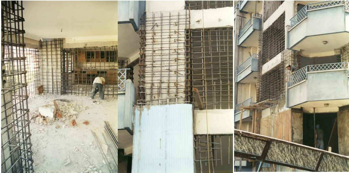
Figure 9.4 Addition of shear walls and frame column jacketing
