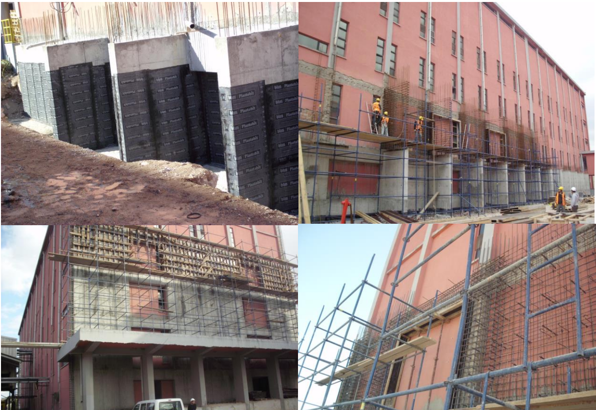
Figure 9.9 Various stages of construction
