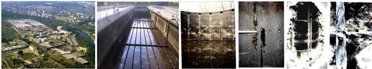
Figure 7.4 Assessment and rehabilitation of large scale prestressed concrete basins and tanks in an urban sewage-treatment plant
